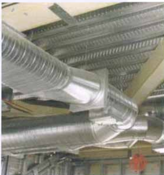
Two Gripple Assemblies & Strut Support
